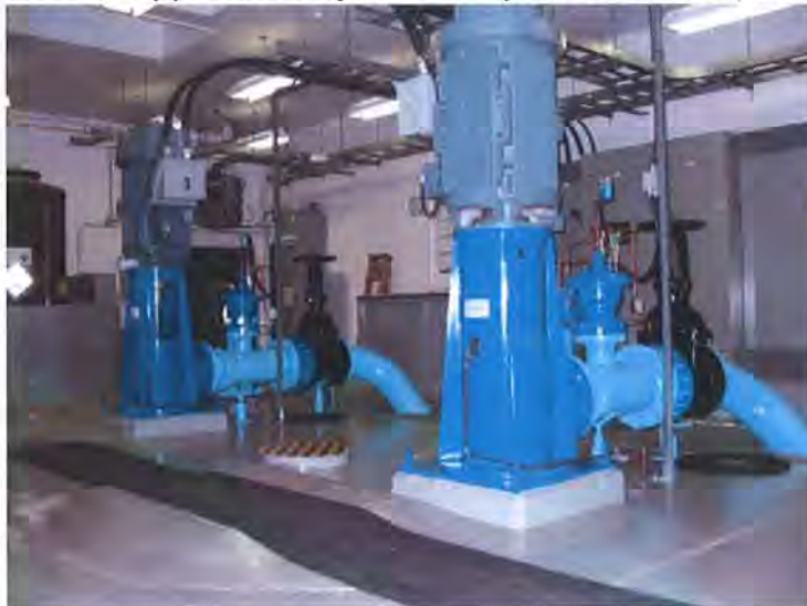
Figure 4 - Zone 1 Pumping Station Canoe
