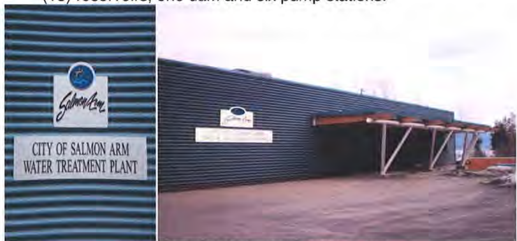
Figure 1 – Water Treatment Plant in Salmon Arm
