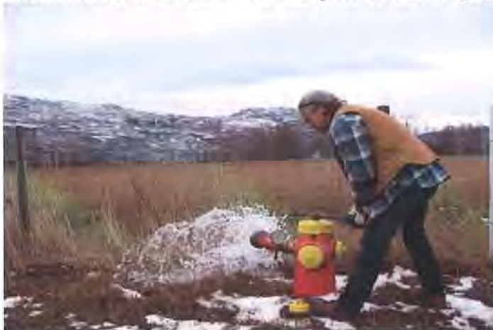
Figure 8 – Utilities Department operator flushing water main as part of regular maintenance
