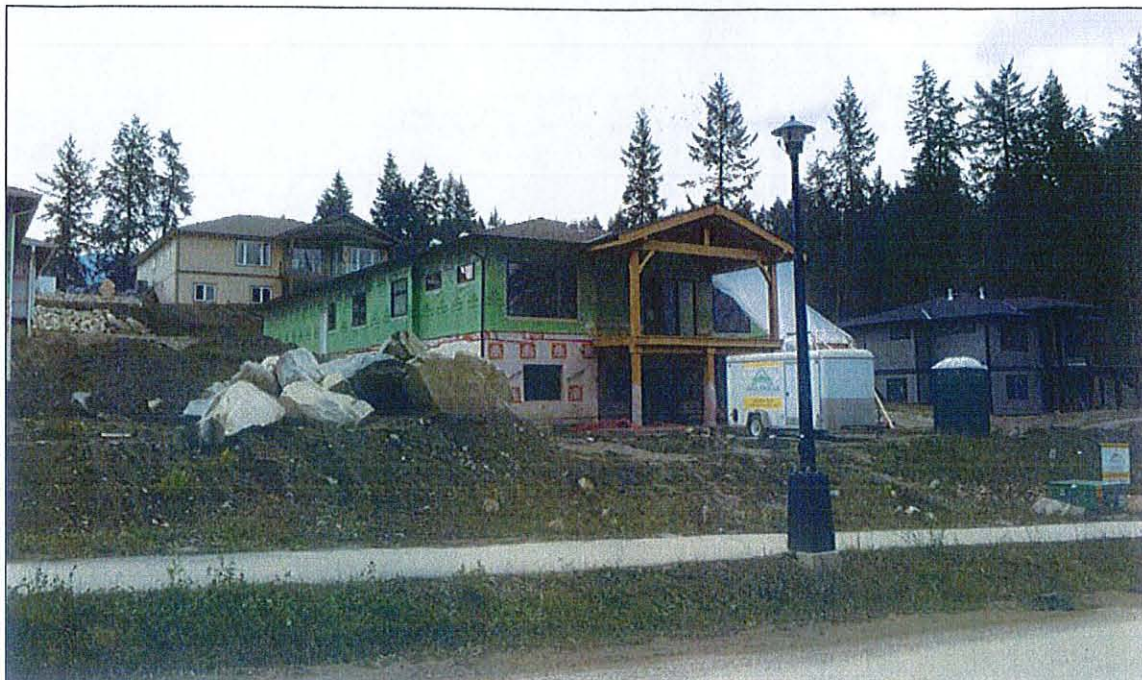
View south-east of subject parcel, showing adjacent development.
