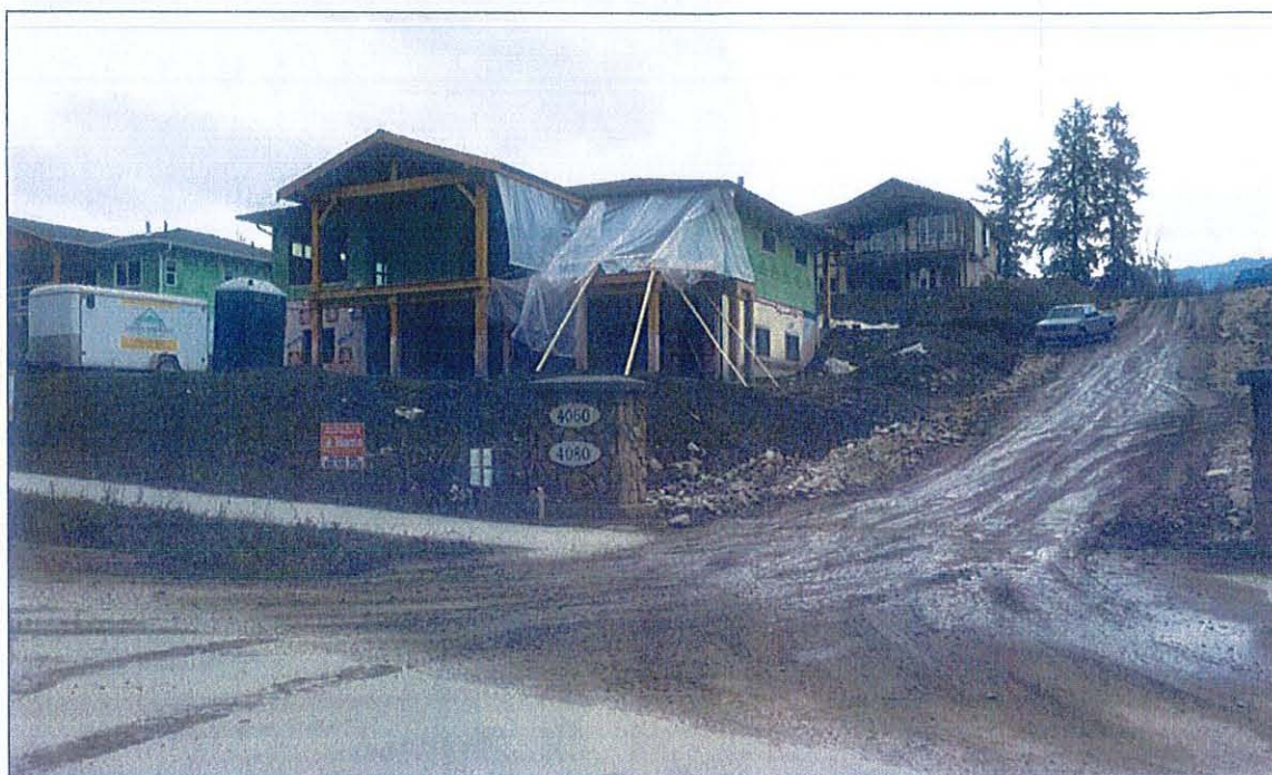
View north-east of subject parcel, showing adjacent development.
