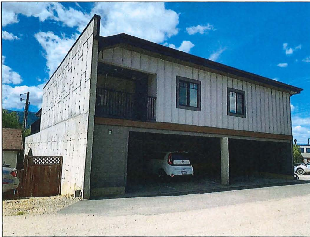
View of subject property looking northwesterly (from laneway)
