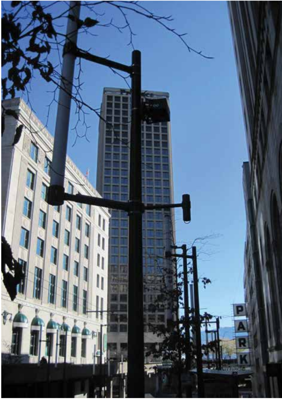
Small cell attachments to decorative street lights (the white vertical element is the light)
