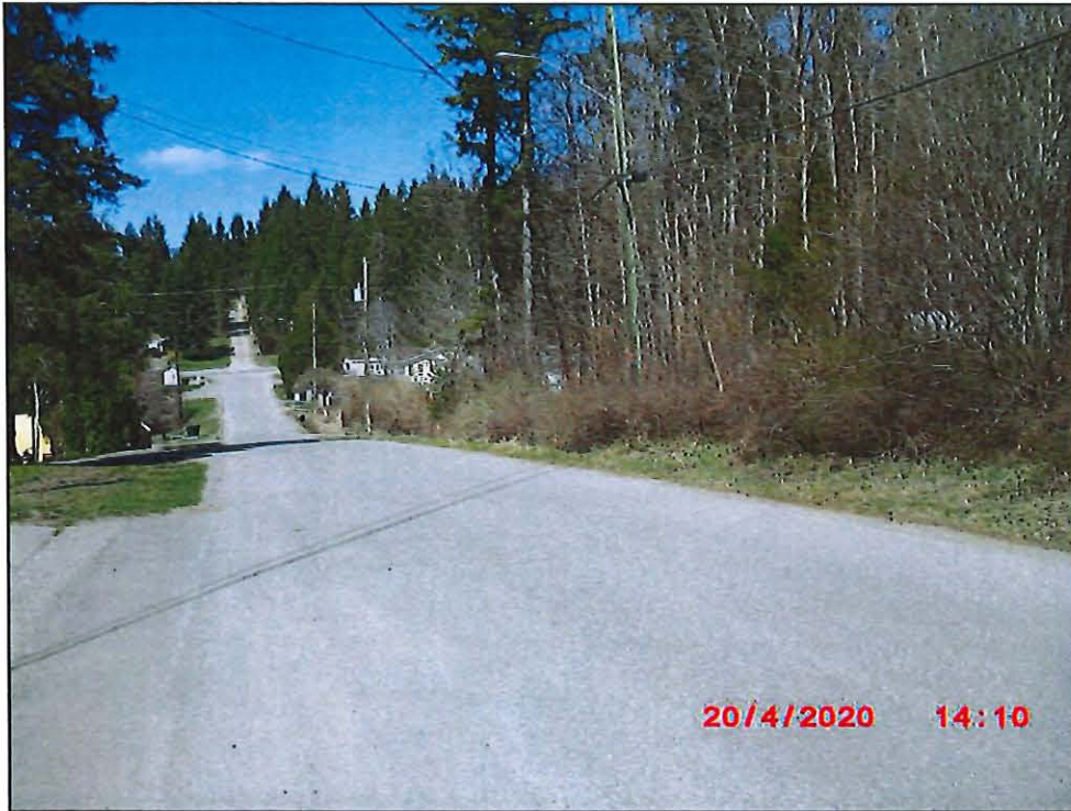
11 Street SE Looking North
