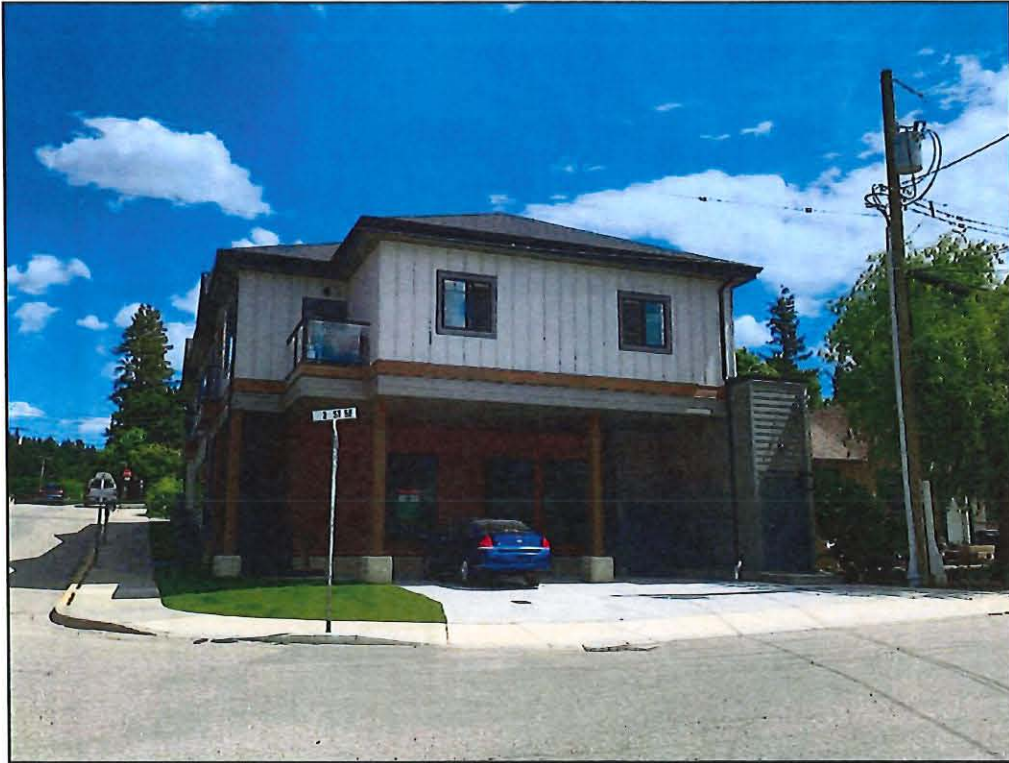
View of subject property looking east (from 2 nd Street SE)
