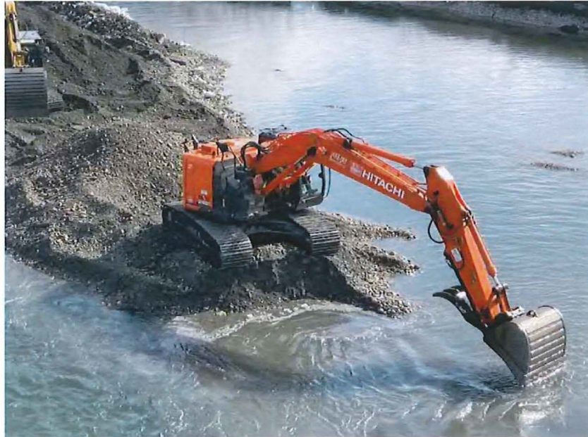
In March 2022, BC Hydro removed about 68,000 cubic metres of gravel from the mouth of the Illecillewaet River, where it flows into Arrow Lakes Reservoir in Revelstoke. The dredging project is part of a tri-party agreement with the Province and the City of Revelstoke. BC Hydro periodically removes accumulated river gravel and excavates a deep channel in the river to reduce the risk of winter ice jams that can cause flooding to low-lying residences. Photo courtesy of Jen Walker-Larsen
