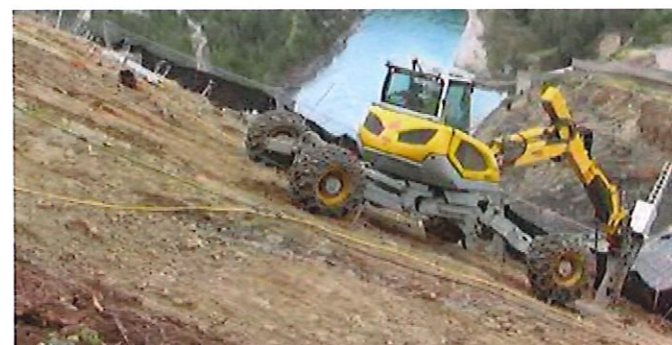
Tethered cat installing anchors.
