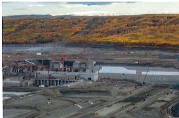
A view of the Site C dam core trench, dam buttress, powerhouse, spillways, and the operational substation in the background.
