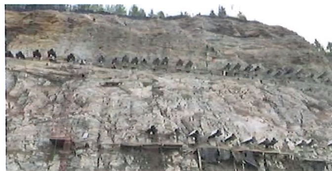
Installing protection for anchors.
