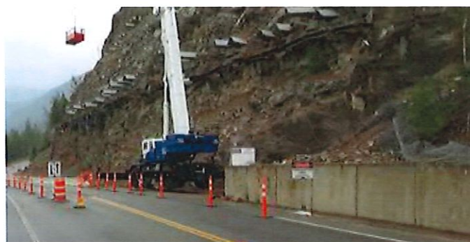
Crane being used to access the slope.
