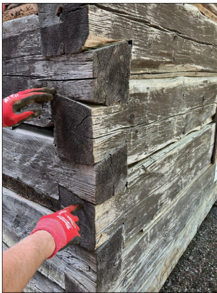
Hand-hewn square log construction with half dovetail joints, circa 2024
