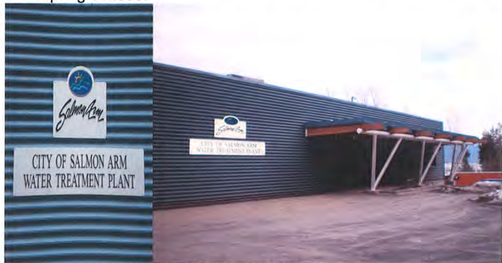
Figure 1 – Water Treatment Plant in Salmon Arm
