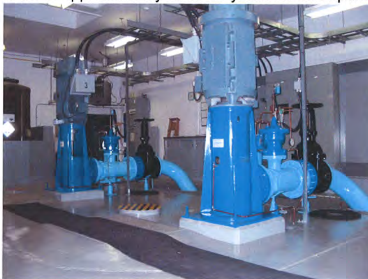
Figure 4 - Zone 1 Pumping Station Canoe
