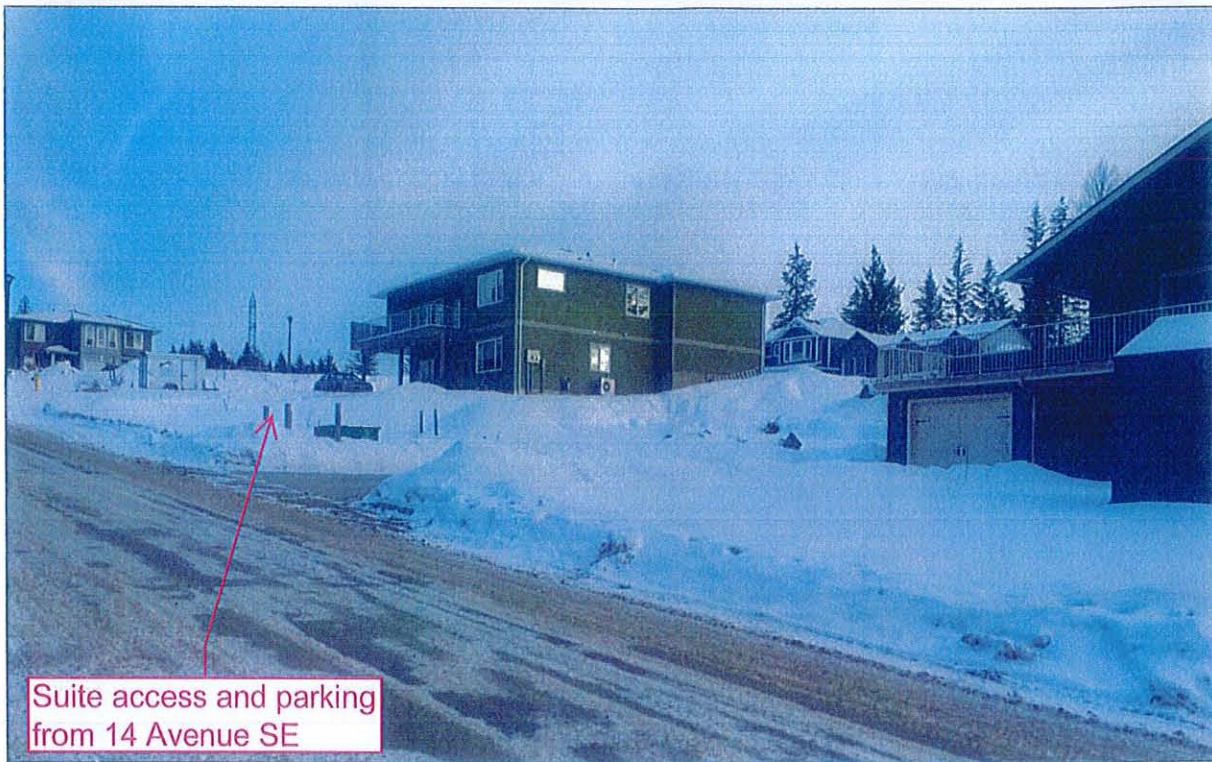
View southeast of the subject parcels from 14 Avenue SE.
