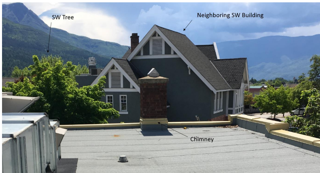
Figure 45: Art Centre South West Roof Shading Obstructions
