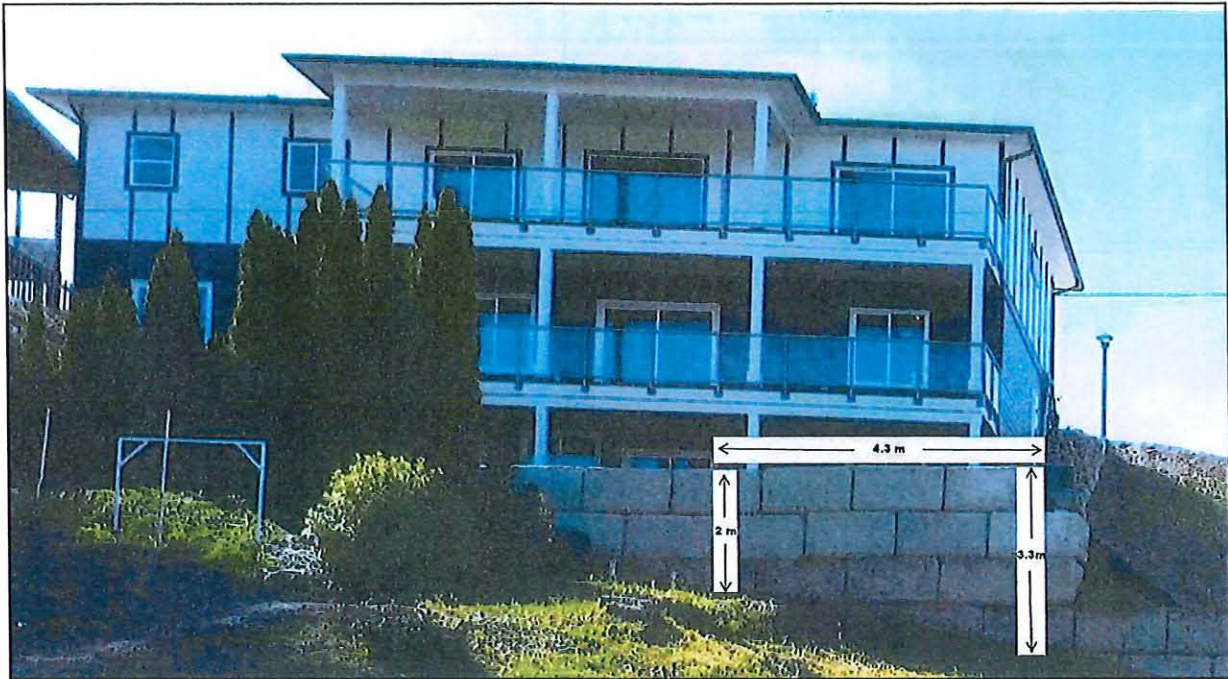
Approximately 4.3 metres (horizontally) is over the maximum permitted height of 2.0 metres.
