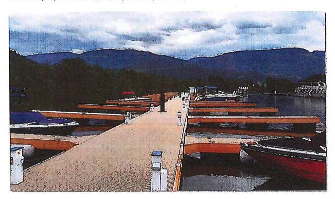
Photo above shows an example of the Landmark Dock System with pedestals including power, water, and LED lighting. This provides the reader with a visual representation of the components to be used for the Salmon Arm Downtown Wharf Marina.
