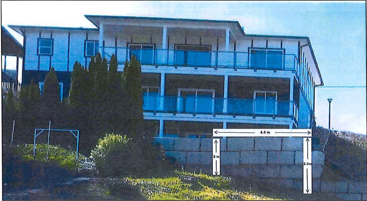
Approximately 4.3 metres over the maximum permitted height of 2.0 metres.
