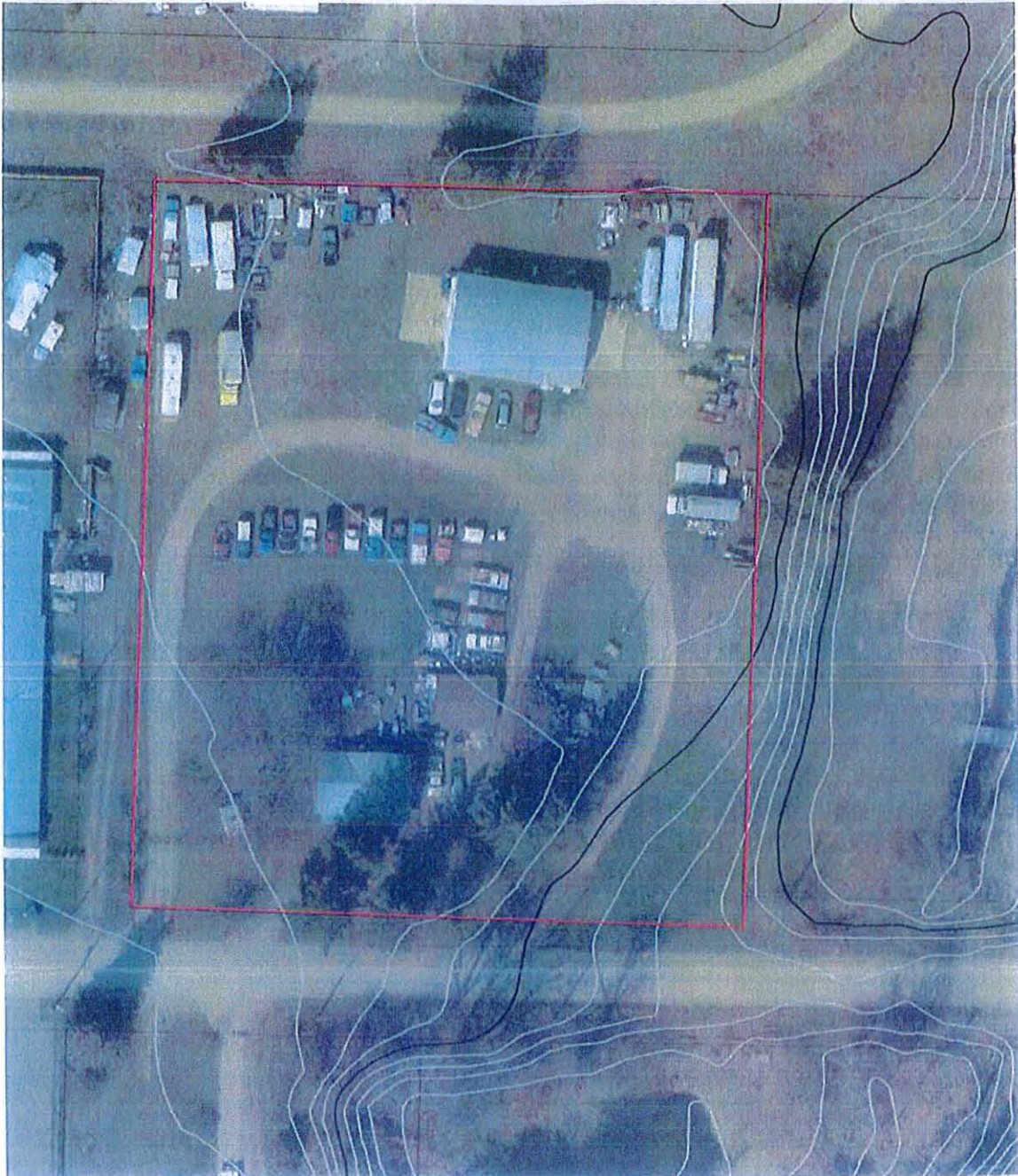
Rough site overview. Parked cars are no longer present. 40x60 shop on north half would stay for the foreseeable future; dilapidated shed and house on south half would be disposed of
