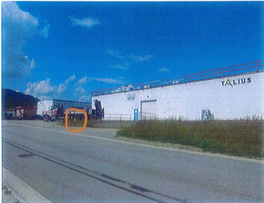
Hydrant on 46 Avenue SE
