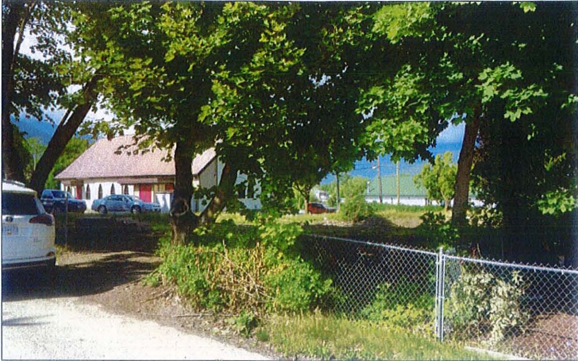
View of subject property looking south-west from lane.
