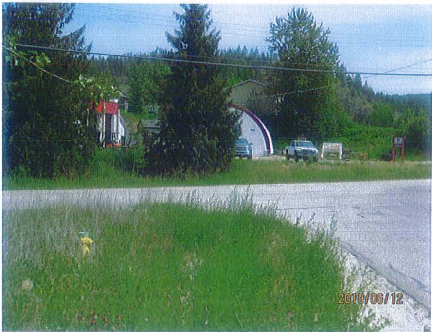
Hydrant at the corner of Auto Road & 46 Avenue SE
