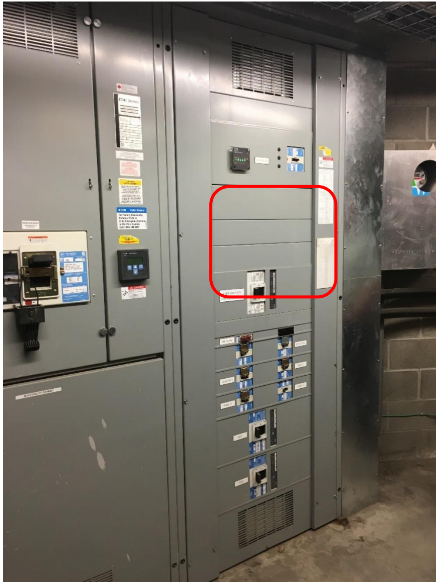
Figure 21: MDC - Room 004 – Spare Breaker Positions
