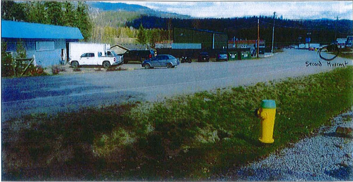
Front of Building; Facing North
