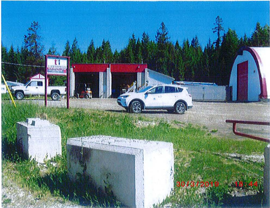
Front of building, facing northwest
