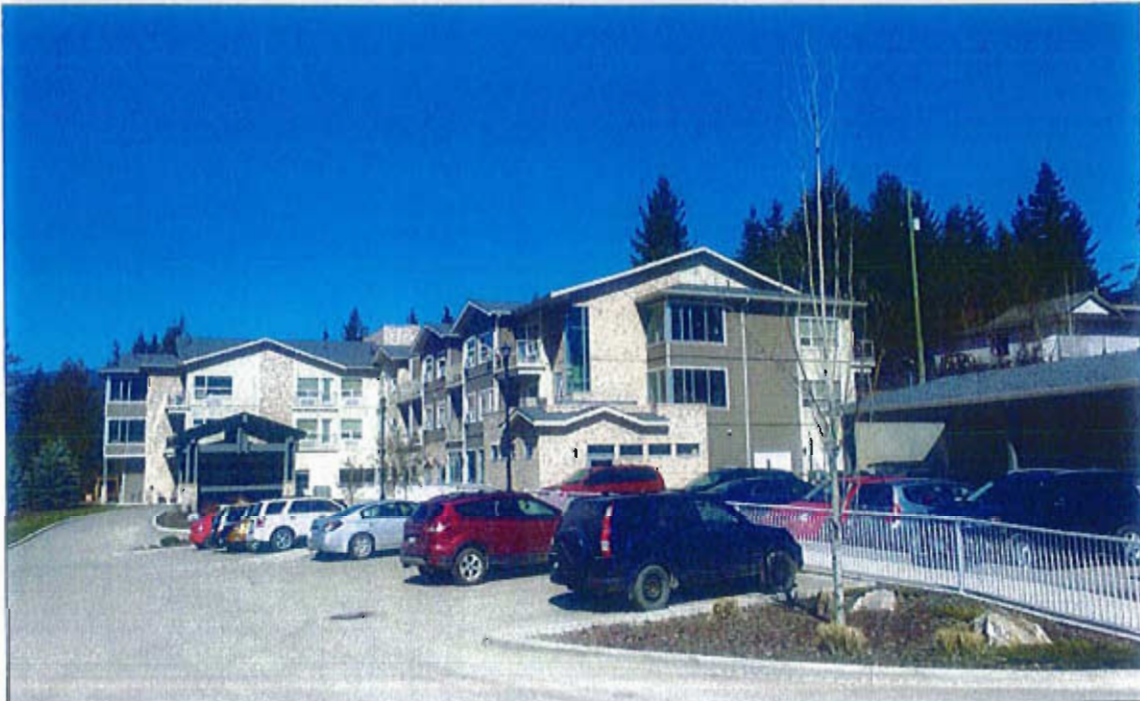
View north of Andover Terrace.
