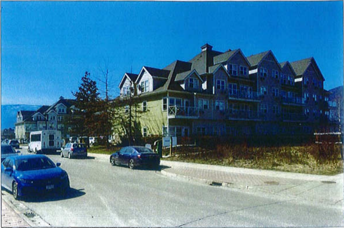
View to the north-west of Lakeshore Manor.
